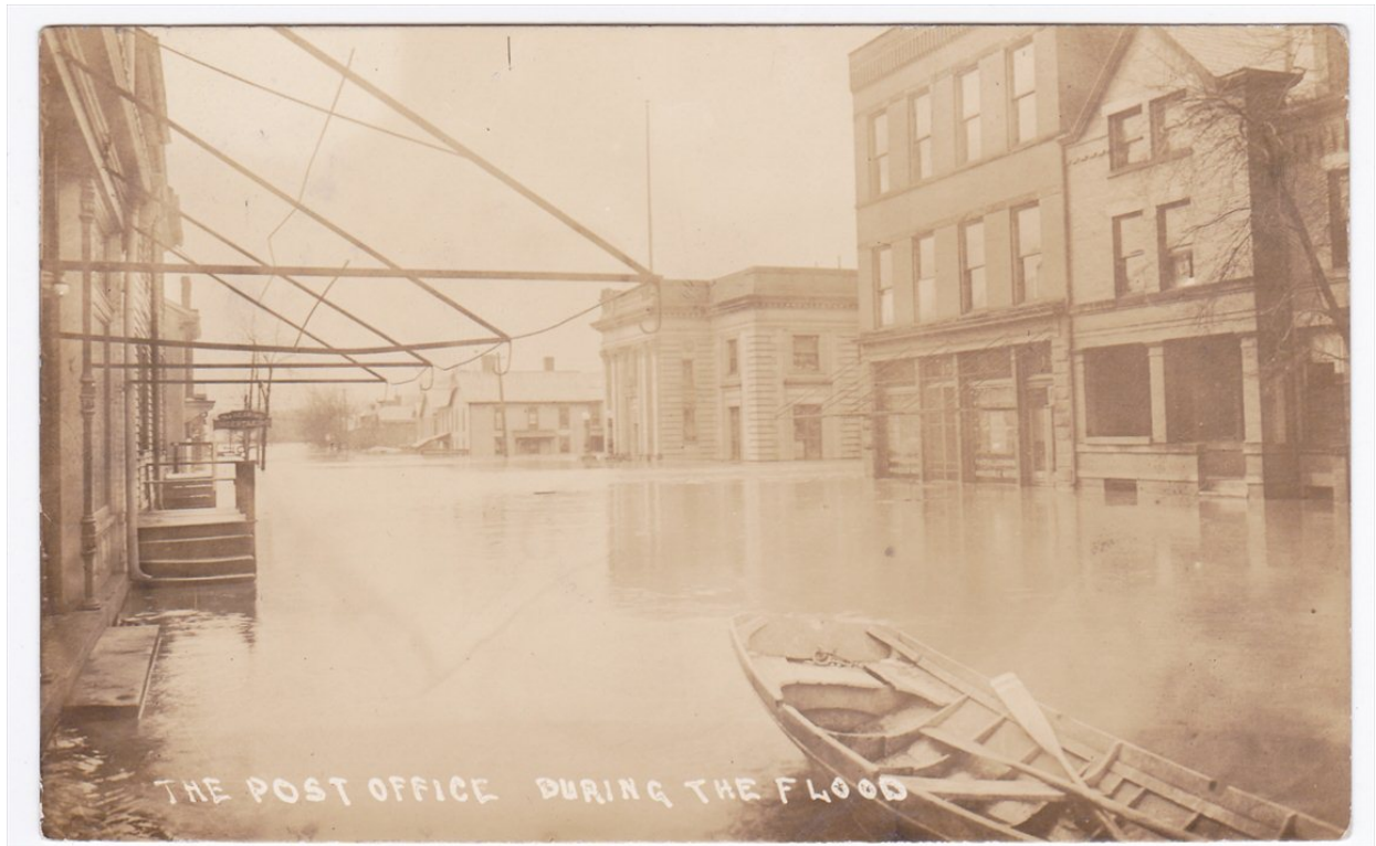
A shot looking south along 5 th Street shows the flood waters receding. The Zanesville Post Office can be seen in the center of the frame with approximately four feet of water around it.
